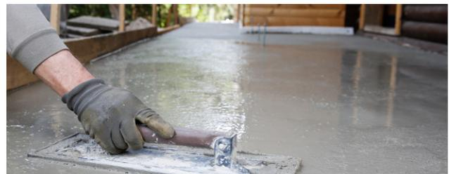
Optimised screed depth and removal of the need to manually mix bagged materials, improves installation time by up to 100%.
